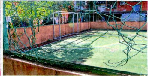
Many of the facilities cannot be used as they are in a state of disrepair.
